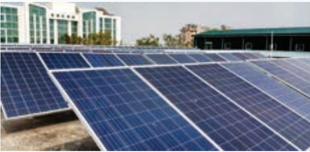
Solar panel, capacity of 100kv installed on the roof top of the main building, Solar street lights
